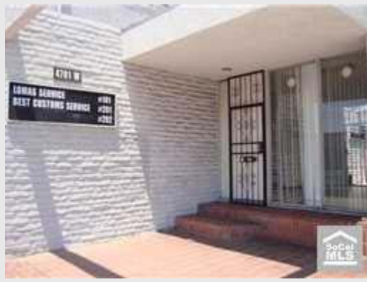
Office Front Entrance
