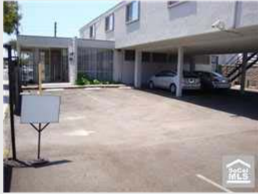
Back Parking Lot
